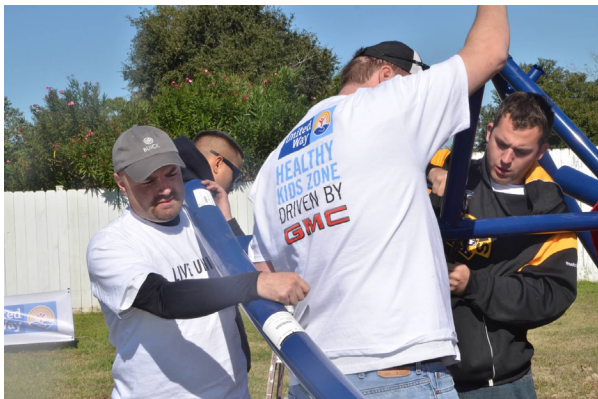
GMC teamed up with United Way to rebuild the Gatto Playground in Gentilly. Volunteers installed a United Way Healthy Kids Zone as part of United Way’s nationwide effort to get 1.9 million more kids active and healthy by 2018.
